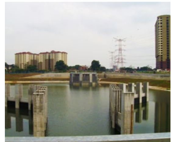
Intakes for the SMART system can draw millions of cubic meters of floodwater into a massive underground tunnel, sparing the streets above from crippling floods.
